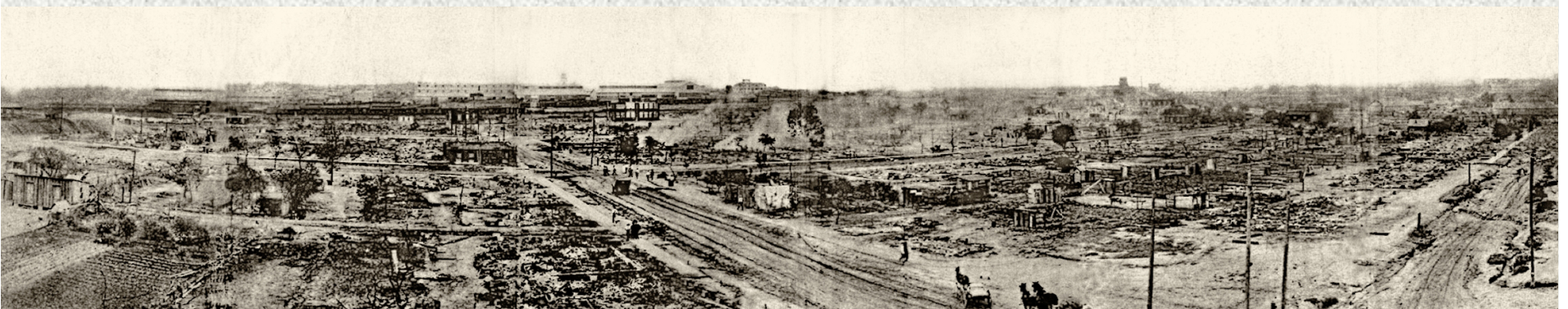
Greenwood neighborhood in Tulsa, May 1921
