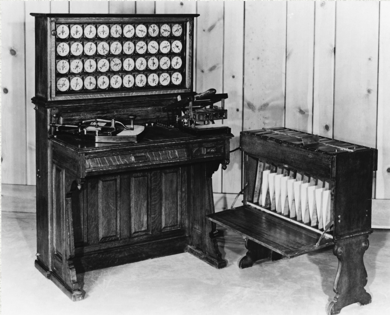
Hollerith electromechanical counting machine, developed for 1890 census, used punchcards to tabulate data. The Hollerith Company later became International Business Machines (IBM, 1924)
