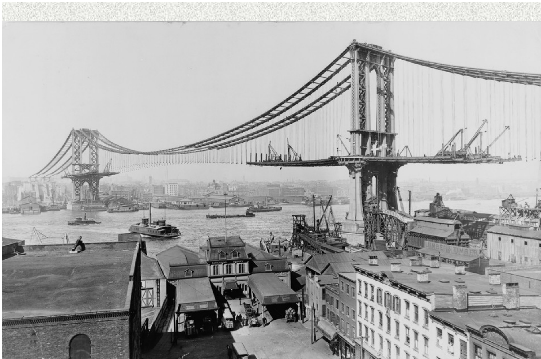
Manhattan Bridge, completed in 1909, same year as the Queensboro Bridge.
